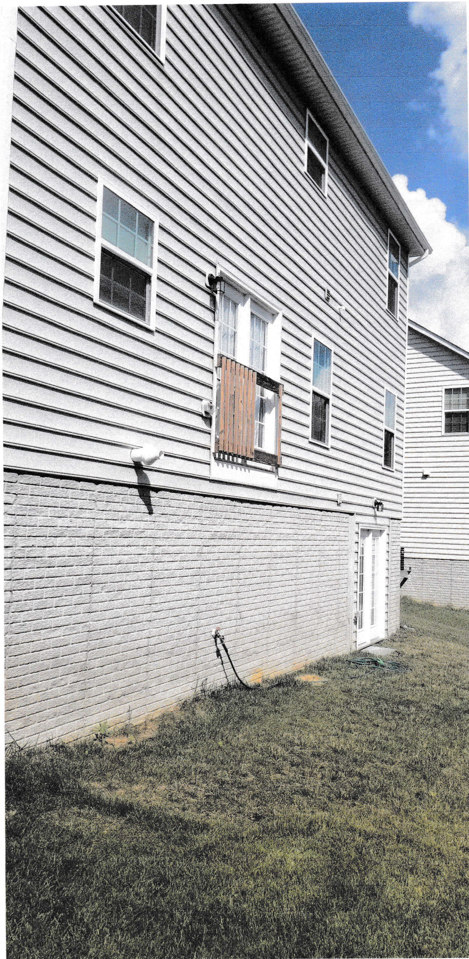
Rear / left side view of property: 1021 Cook Dr. SE
